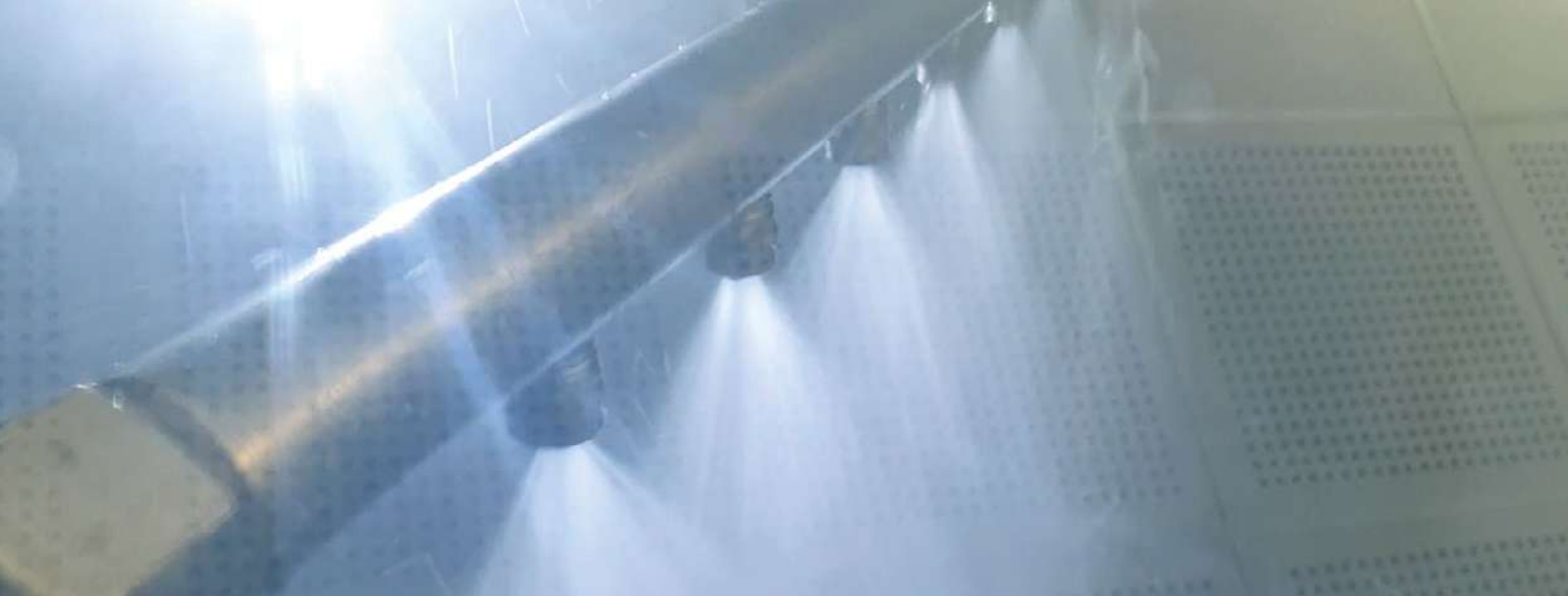
Mechanical cleaning in the HTW
