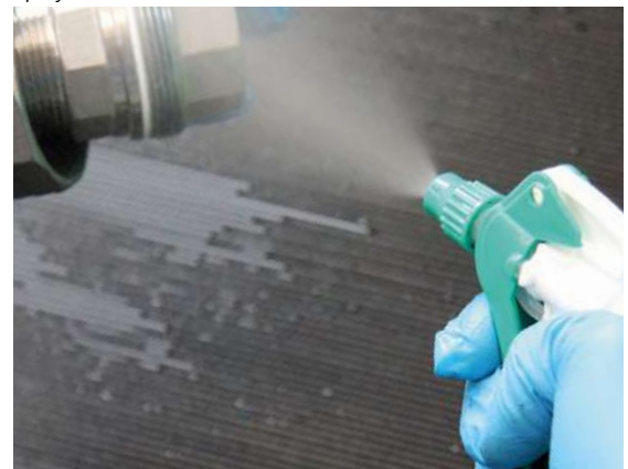
Spray on GS 200 – remove sealant
