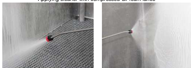
Applying cleaner with compressed-air foam lance
